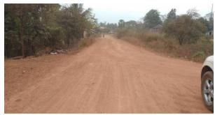
7. The road will be upgraded to a DBST and RC road along the existing road alignment with a proposed road base-width that ranges from 10.0 to 18.0 meters and with a total length of 11,231 meters.
