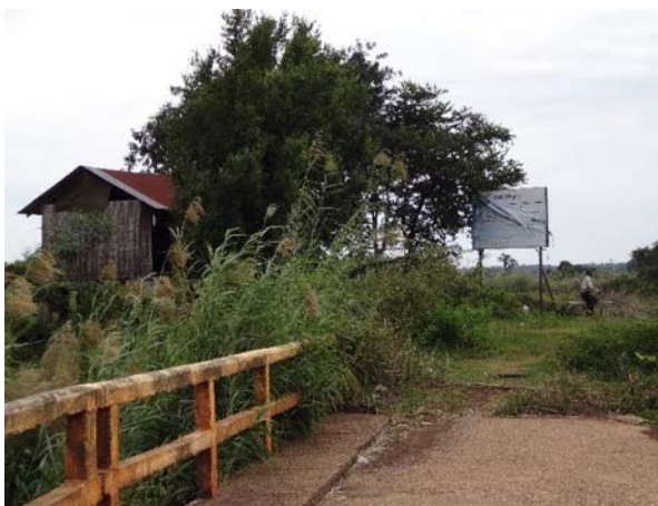
Photo from the bridge (the 1 st house)
